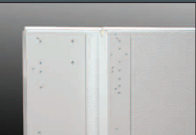
White painted end stiles are 4" to 8" wide to accommodate double or single-end hinges.
